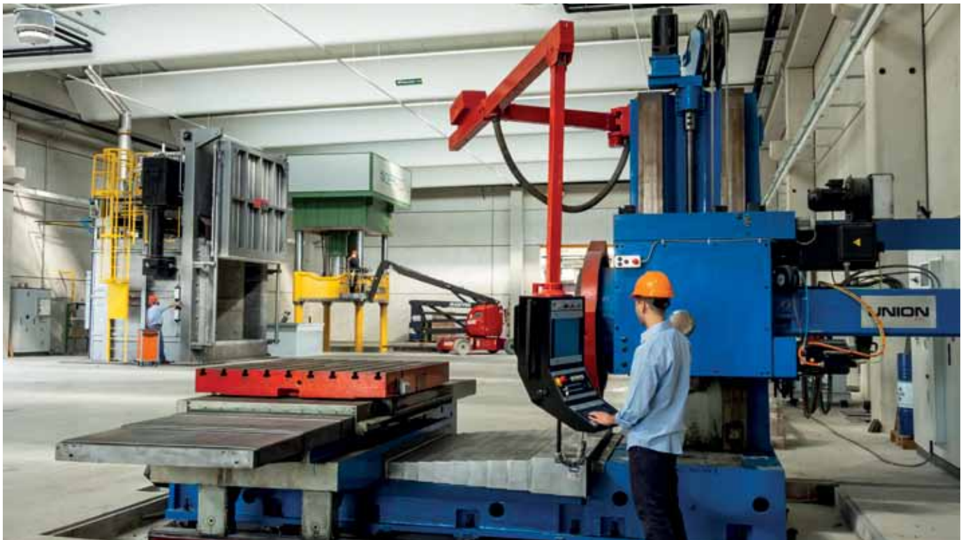
The new furnace, pressing and boring machines
